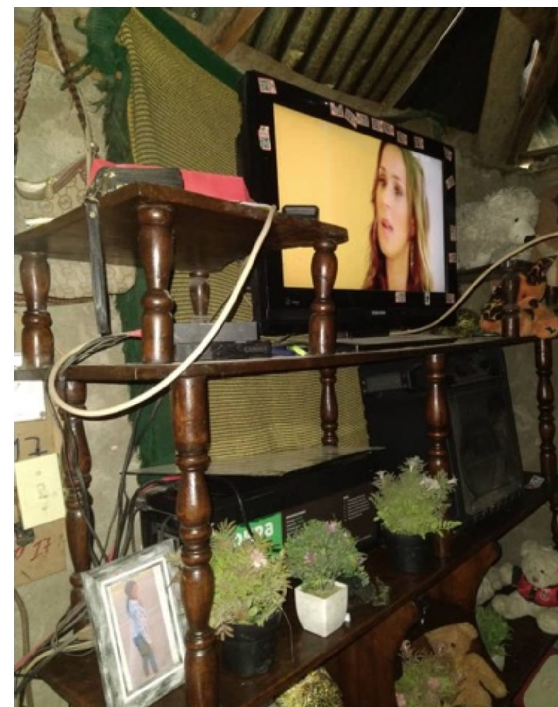
Photo Battery in the living room of one of Alina Enèji's customers.
