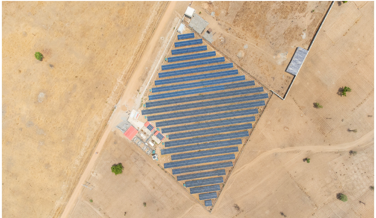
Zawaciki IMG generation plant.
