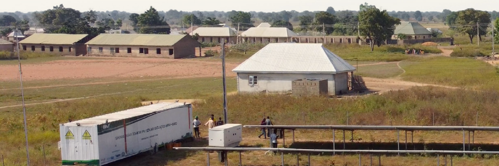
A solar mini grid providing clean, reliable energy for the Shimankar community in Nigeria. Photo: Global Energy Alliance
